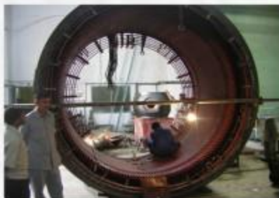
8MW,11KV STATOR REWIND (AT SITE)
