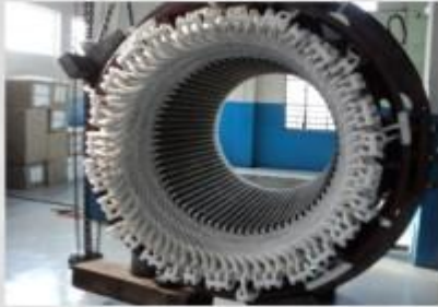
8 MW, 11 KV, STATOR REWIND
