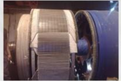
7000 HP DC ARMATURE REWIND (AT SITE)
